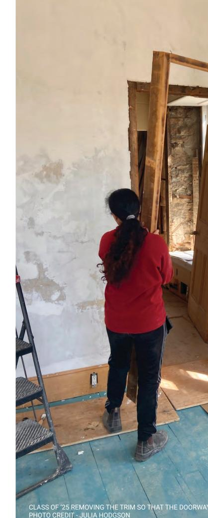
CLASS OF '25 REMOVING THE TRIM SO THAT THE DOORWAY COULD BE FRAMED IN FOR THE FUTURE THIRD FLOOR BATHROOM
